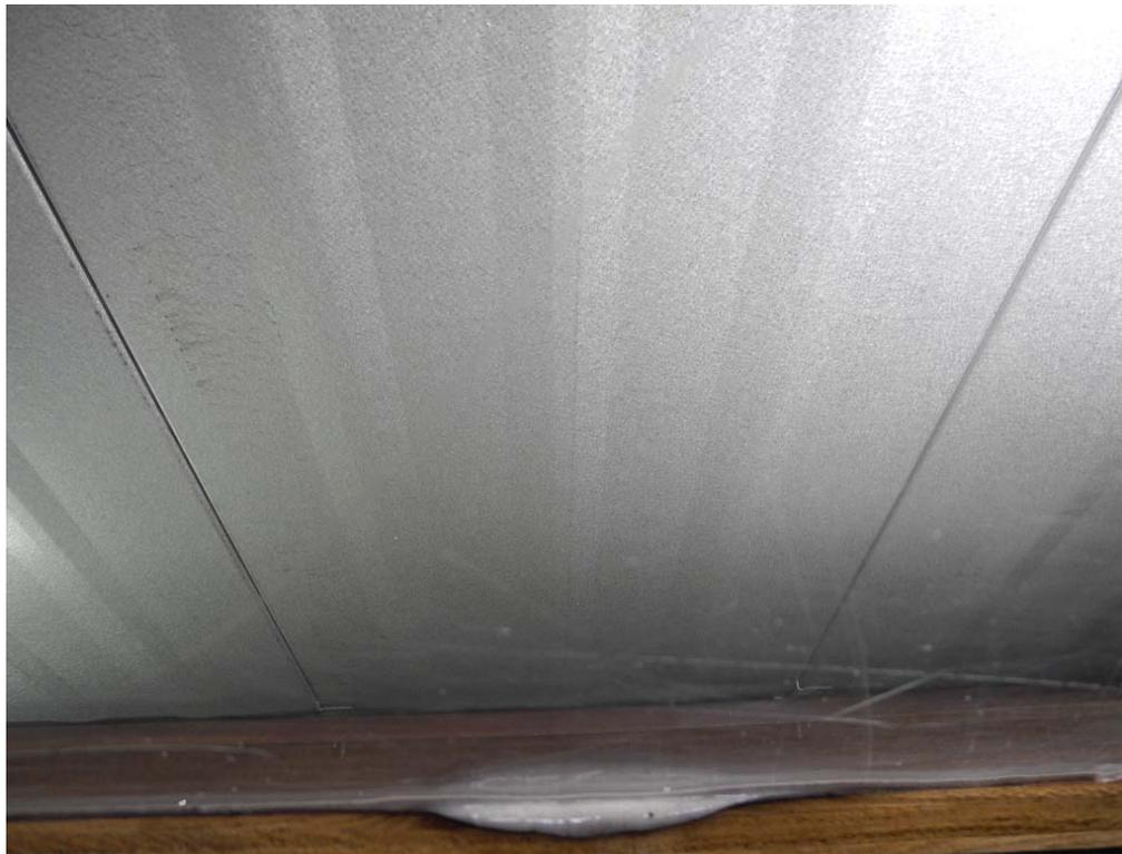
**PHOTO 10** View of panel sidelaps during the water test (DSCN0897)
