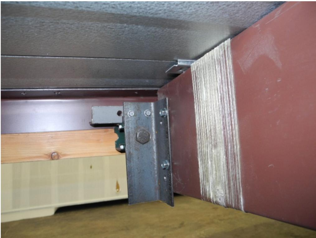
**PHOTO 4** View of support movement to simulate thermal movement of panel.
