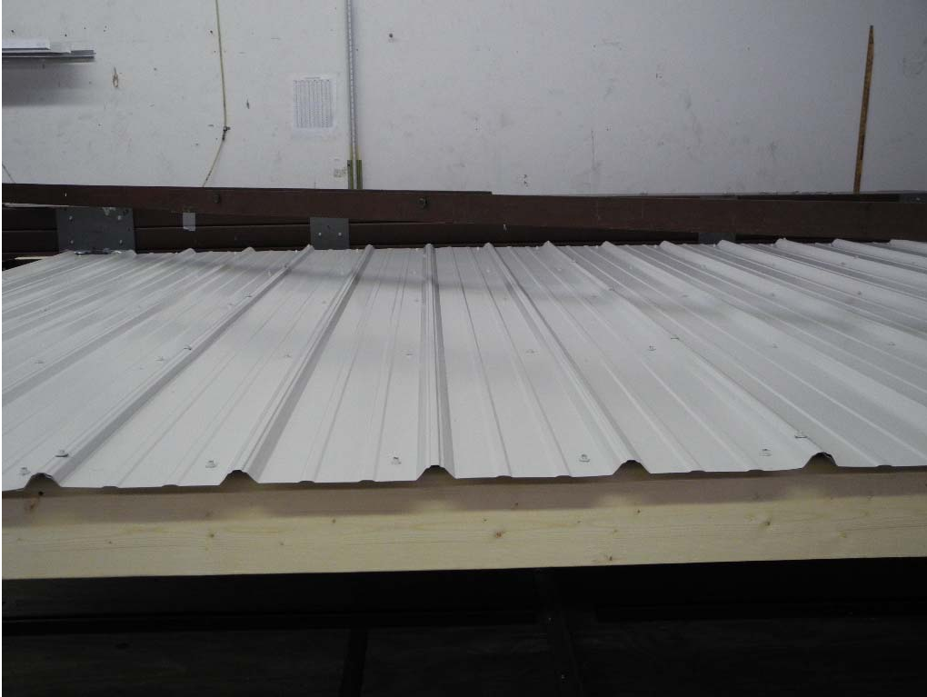
PHOTO 3 View of the panel fasteners at end and interior supports. (DSCN1012)
