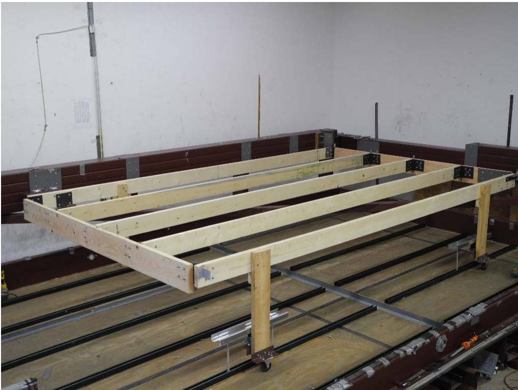
PHOTO 2 View of the wood support layout. (DSCN1040)
