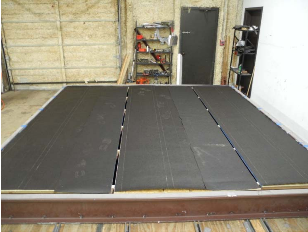
PHOTO 1 View of OSB or plywood deck with felt. (DSCN6734)
